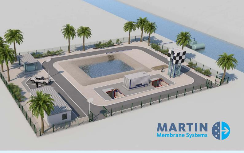
The **Package Plant for drinking water** is a cost-effective compact water plant based on a modernised version of the conventional water treatment processes, which means that all the necessary components for coagulation, flocculation, clarification, filtration and disinfection are combined in a compact system.
